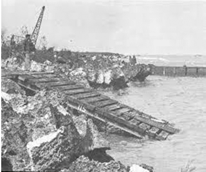
“Doodlebug” landing ramps improvised by the SeeBees for the Tinian Invasion, designed, built, tested and used in just over 2 days
